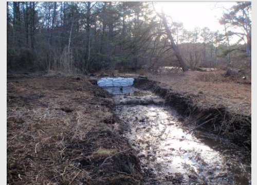
Cleared Northwest Creek (temporary sandbags in place).
