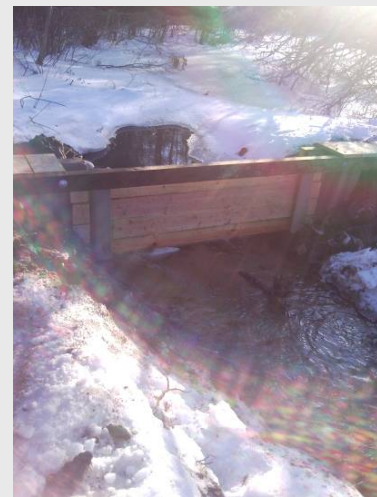
Constructed Weir in Northwest Creek.
