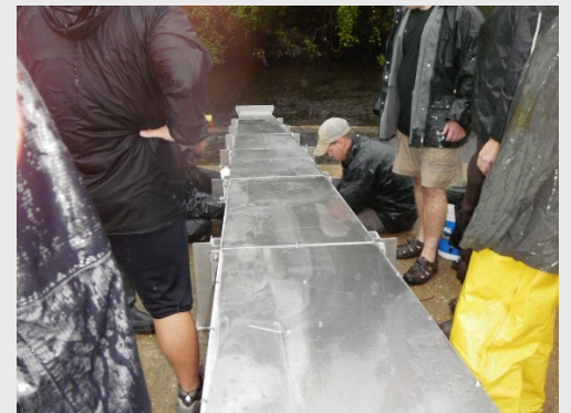
Installation of the middle ladder
