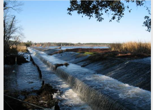
Goose Creek Dam
