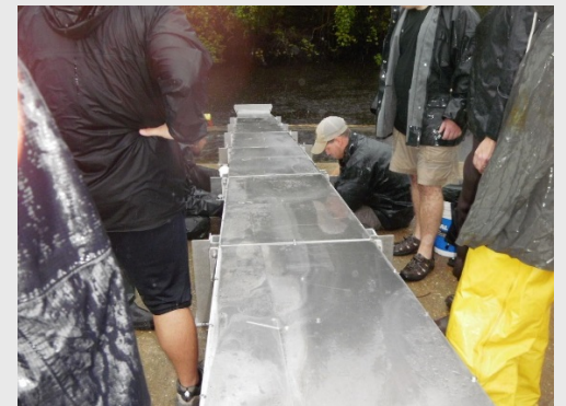
Installation of the middle ladder
