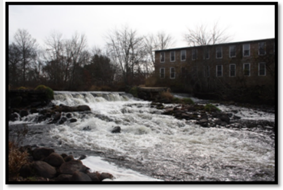
Bradford Dam, Westerly, Rhode Island
