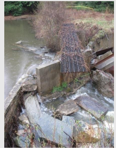
Former dam on Shoreys Brook
