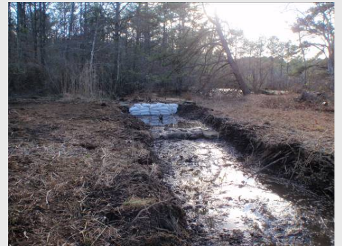
Cleared Northwest Creek (temporary sandbags in place).
