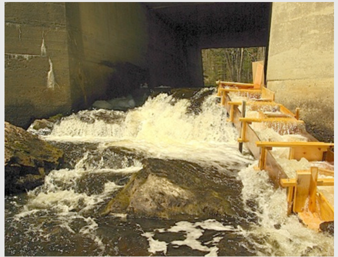
The Route 172 barrier on Patten Stream (facing upstream), with temporary fish ladder in place.
