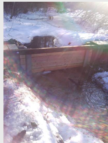
Constructed Weir in Northwest Creek.
