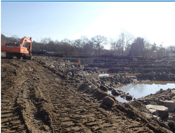
Bradford Construction- weirs with low flow outlets. Photo courtesy of P. Edwards
