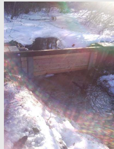
Constructed Weir in Northwest Creek.
