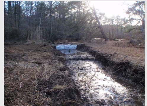
Cleared Northwest Creek (temporary sandbags in place).
