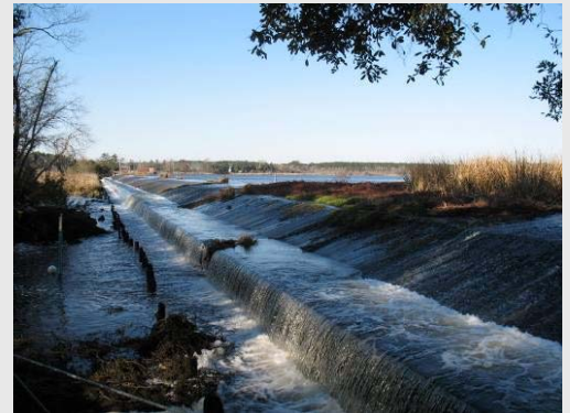
Goose Creek Dam
