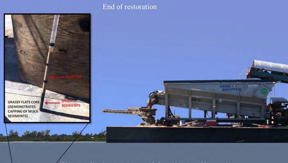
Water quality improves as muck layer is capped by sand and is no longer re-suspended
