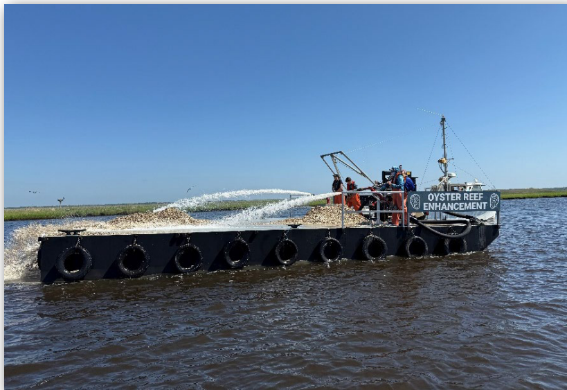
Loose broadcasting of recycled shell using a barge and water cannon. Credit: NJDEP
